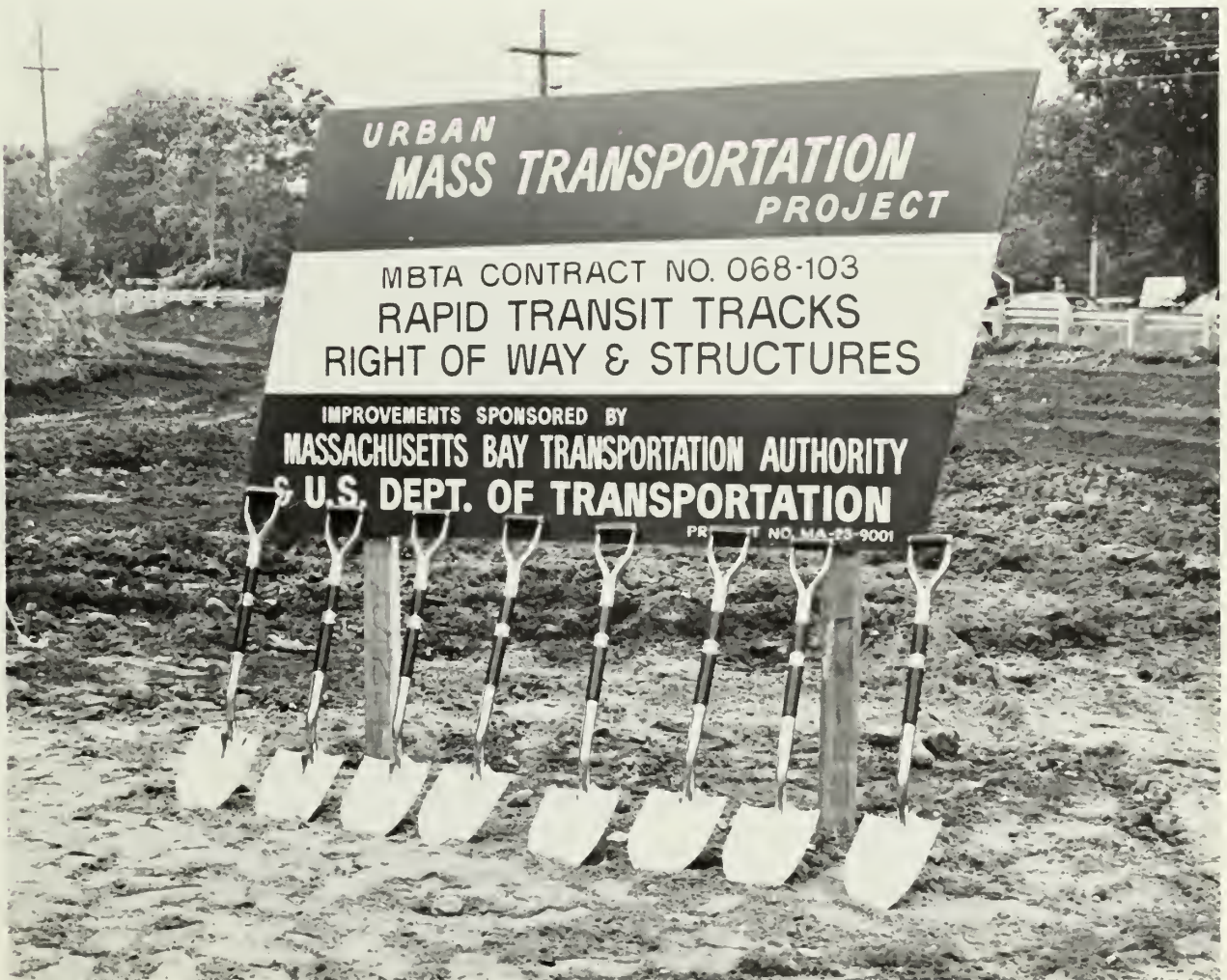
GROUNDBREAKING DAY for the Red Line's new Braintree Station and 1,200-car parking garage was July 13.
